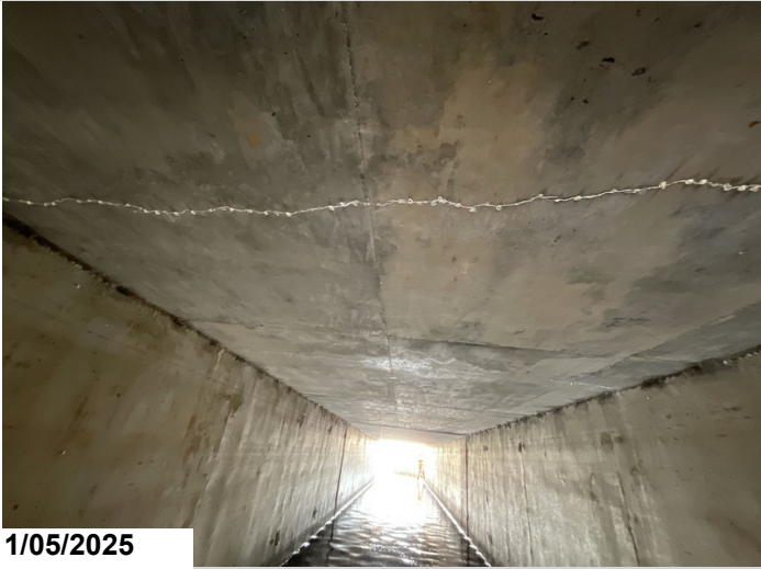
Typical crack with efflorescence. CS2
