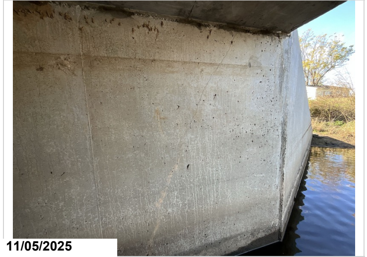
Barrel 1 Left Side Back wall diagonal crack CS3
